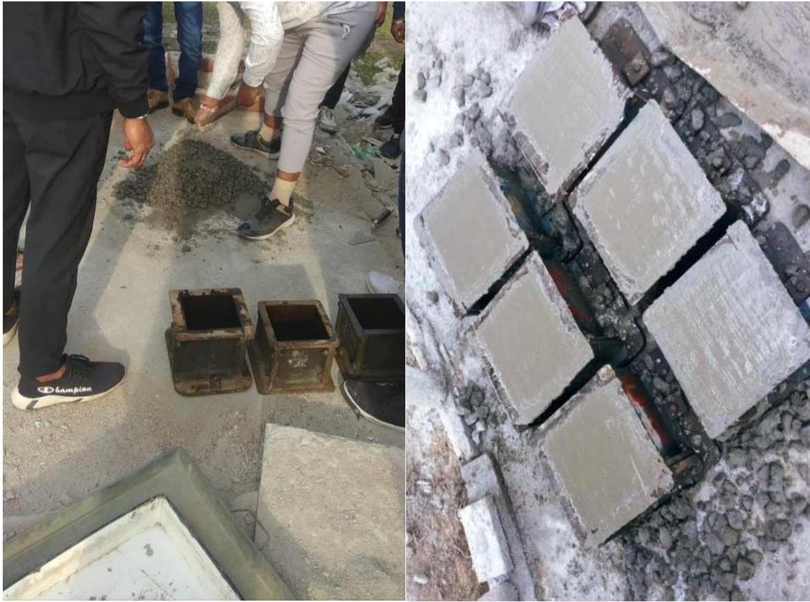
Figure 1i. Casting of cubes
